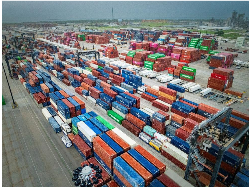
Aerial view of Port Houston's Bayport Container Terminal.
